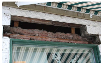
Wide open as new lintel for front window is manufactured
